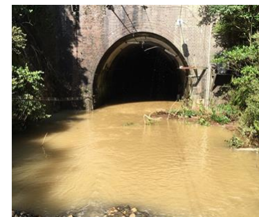
■ Sediment runoff on the Nippo Main Line between Tsukumi Station and Hishiro Station
